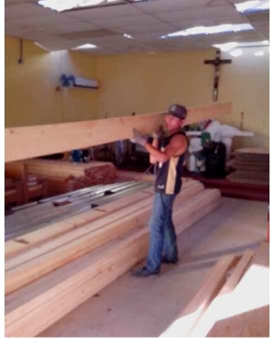
RAMON HELPING TO BUILD
